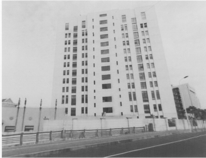
FIGURE 7: Unit 61398 Center Building 208 Datong (rear view, possible generator exhausts visible) Image Copyright 2013 city8.com
